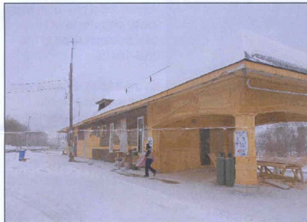
Bradford GO Station undergoing renovation
